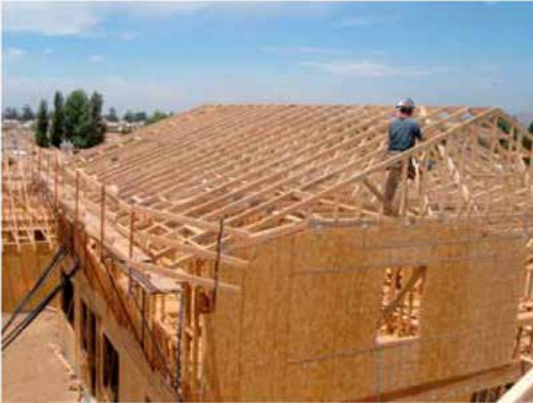
Bracing of gable end truss
