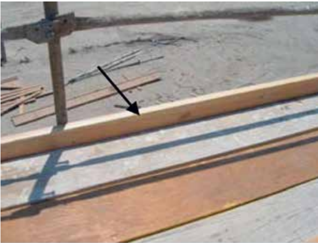
A A 2" x 6" toeboard is required when the scaffold is used as an edge protection device.
